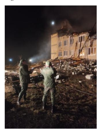
In the evening of April 19, 2021 structures of a three-storey residential building in Margusha village of Nizhny Novgorod Region collapsed resulting in partial collapse of the ceiling of the second and the third floor.
